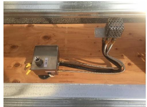
8. With every fire feature an orifice must be installed between the outlet of the Ignition Control Box and the burner. When the fuel type is Natural Gas a Natural Gas Orifice is to be installed. When the fuel type is Propane a LP Air Mixer Orifice is to be installed. The noticeable difference between these two orifices are the 6 Air Holes in the LP Air Mixer orifice.
